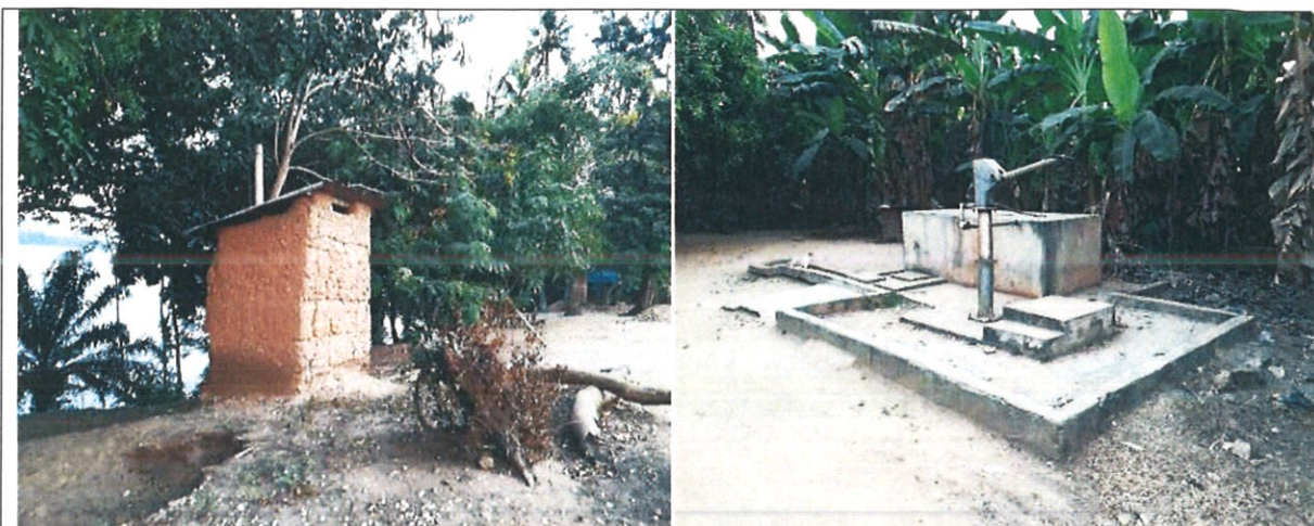
Photograph 2- 2: A household toilet facility at Volivo
